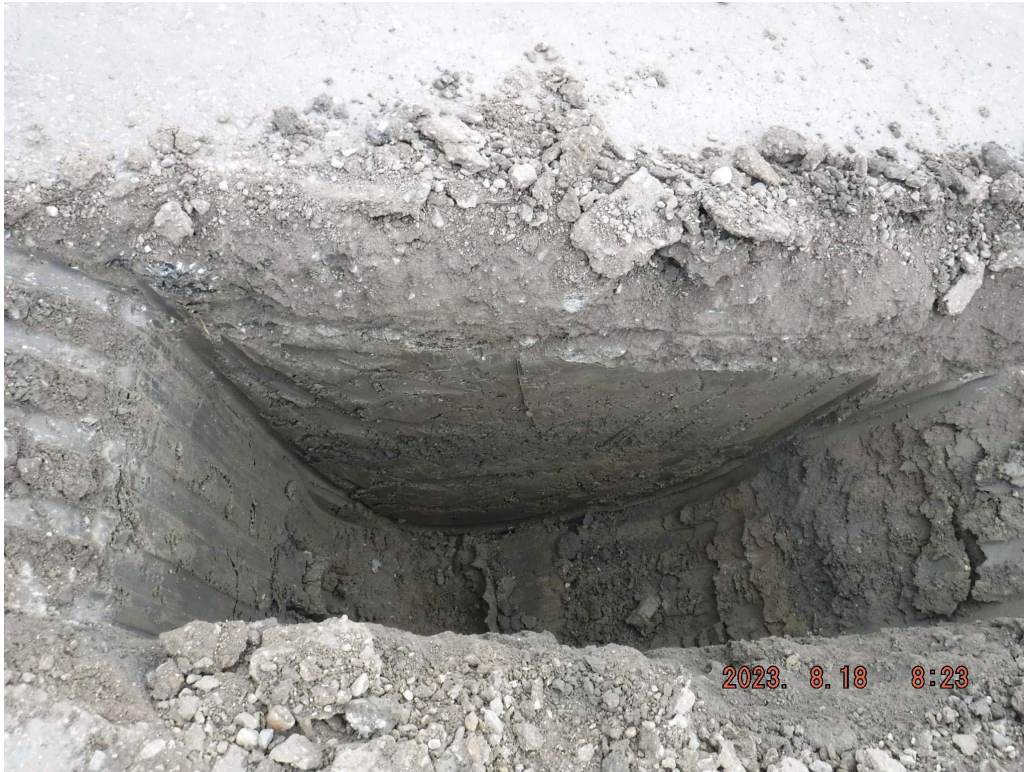
Photograph 1: Looking at TP23-1
