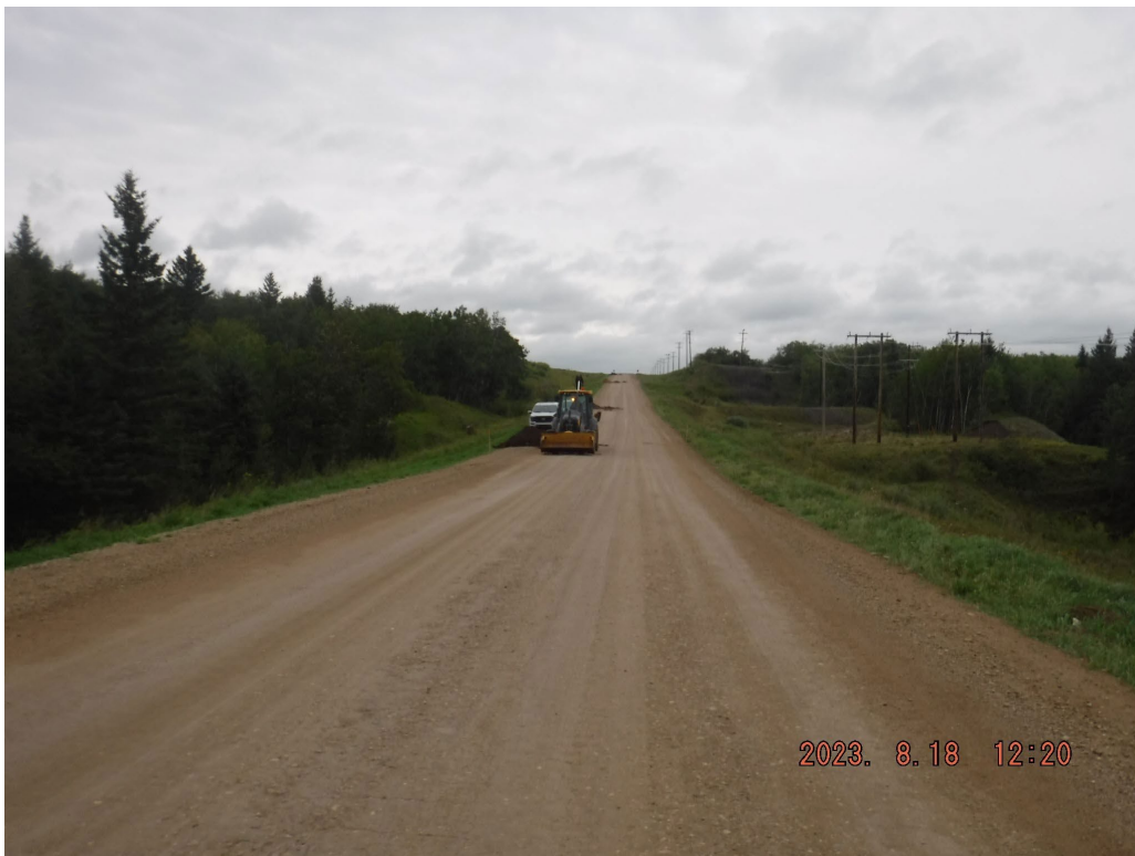
Photograph 4: Looking east at TP23-4
