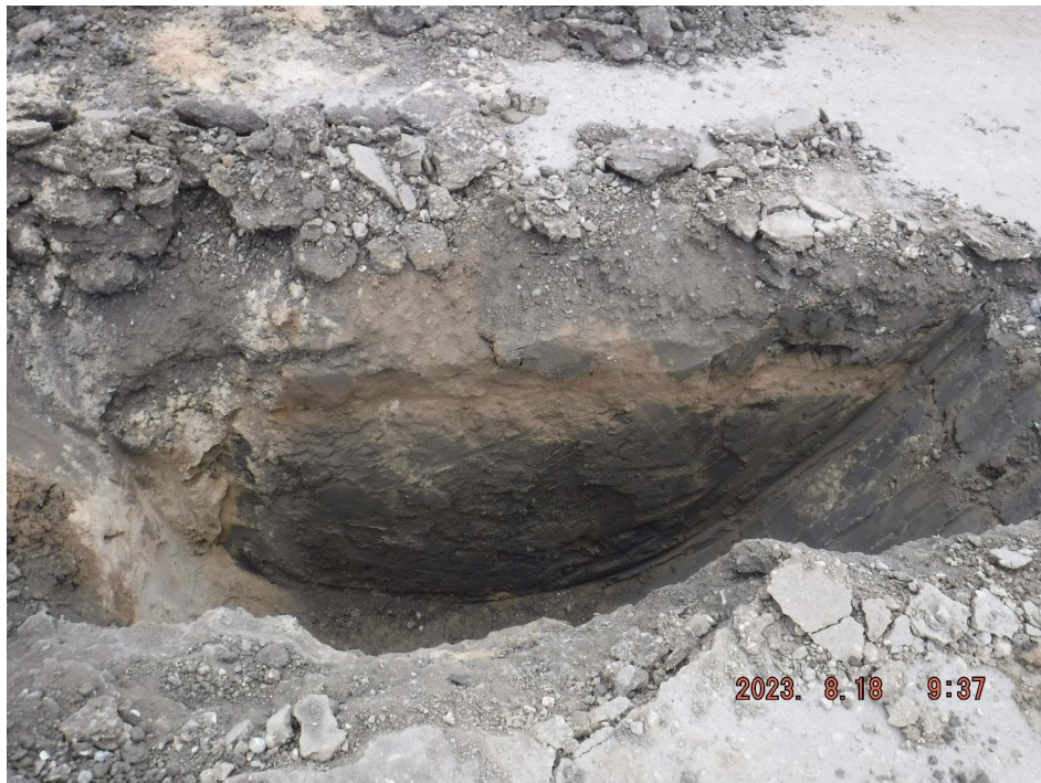
Photograph 2: Looking at TP23-2 east wall
