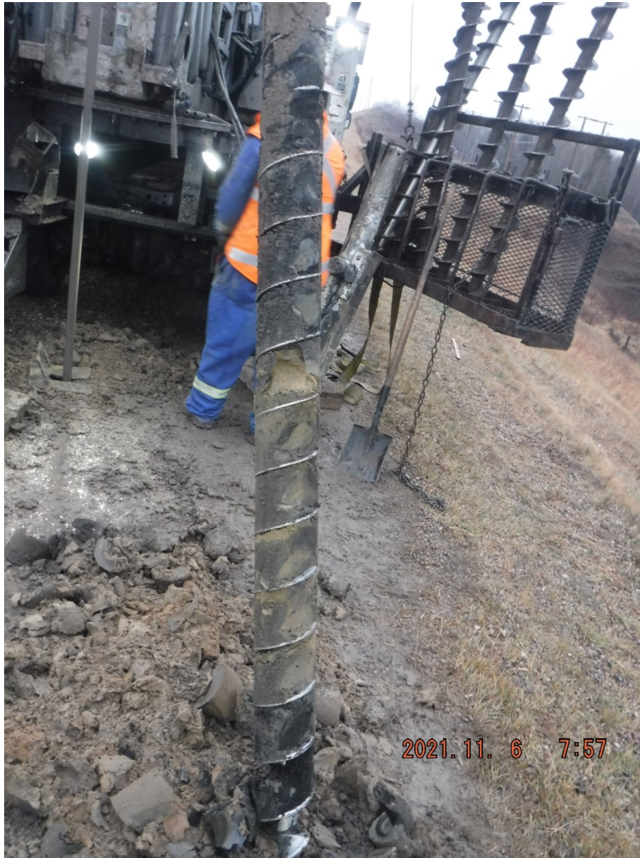
Photograph 5: Buried topsoil, BH21-4 at a depth between 8 and 10 m
