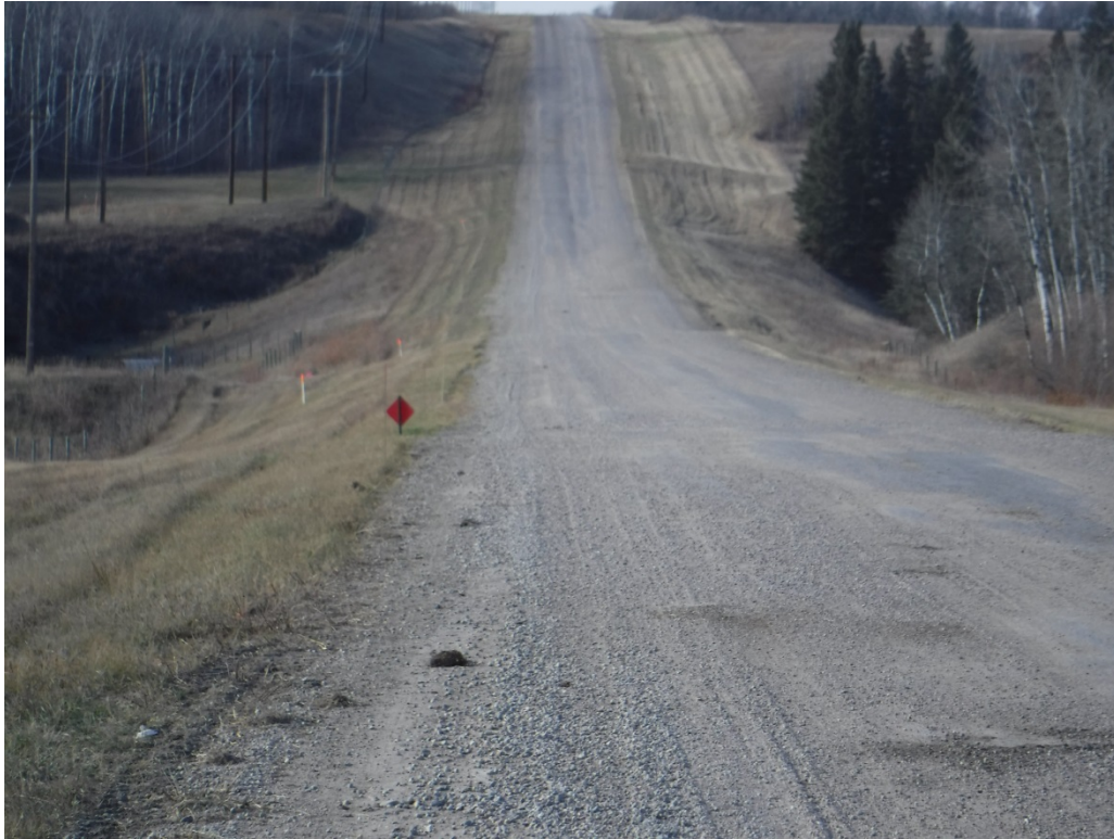
Photograph 3: Looking west along the alignment
