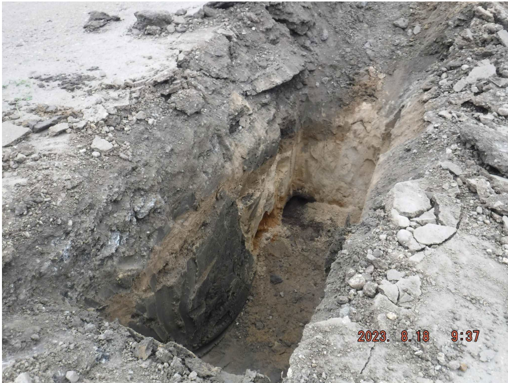
Photograph 3: Looking at TP23-2 west wall
